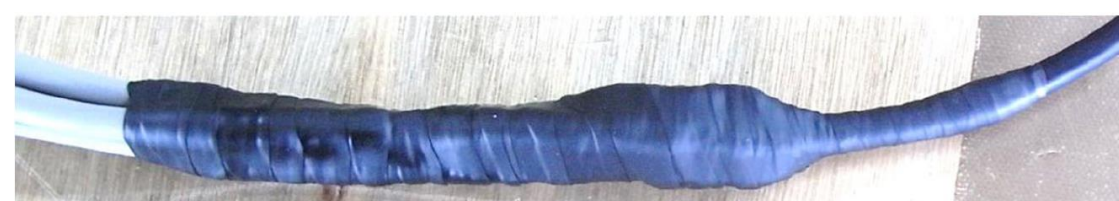
図14.防水処理(参考)/FIG 14. Waterproof treatment (reference)
