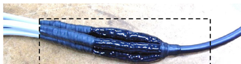
図13.防水処理(参考)/FIG 13. Waterproof treatment (reference)
