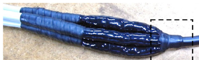
図12.防水処理(参考)/FIG 12. Waterproof treatment (reference)
