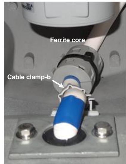
14) Clamp the cable by the cable clamp-b.
